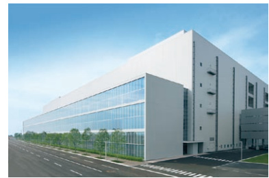
Solar cell plant at GREEN FRONT SAKAI
