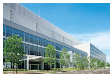
LCD panel plant at GREEN FRONT SAKAI
