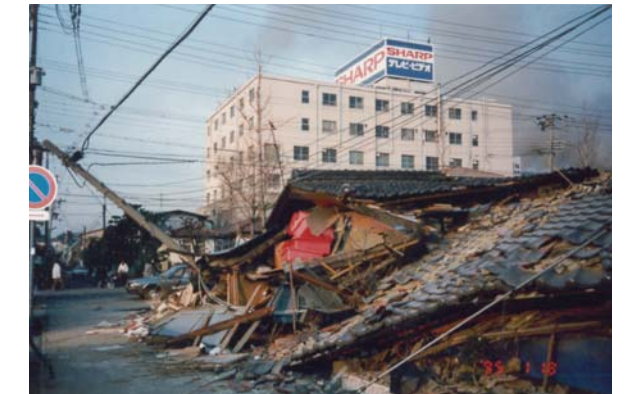
Devastation around the Sharp Kobe Building
